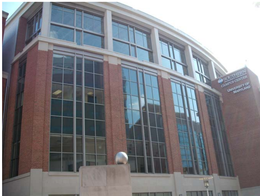
Figure 39: Building Façade Close-Up
